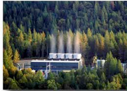
Photo of Geysers Geothermal Power Plant courtesy of Calpine
